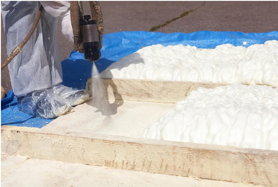
Polyurethane roof insulation
