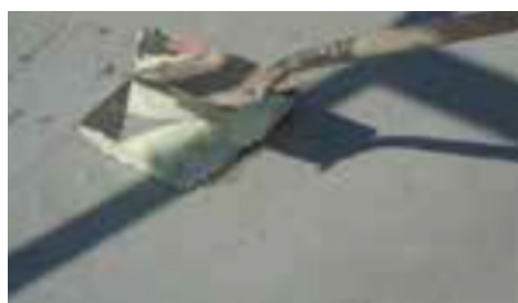
Fig. 4-4 Bond Failure
